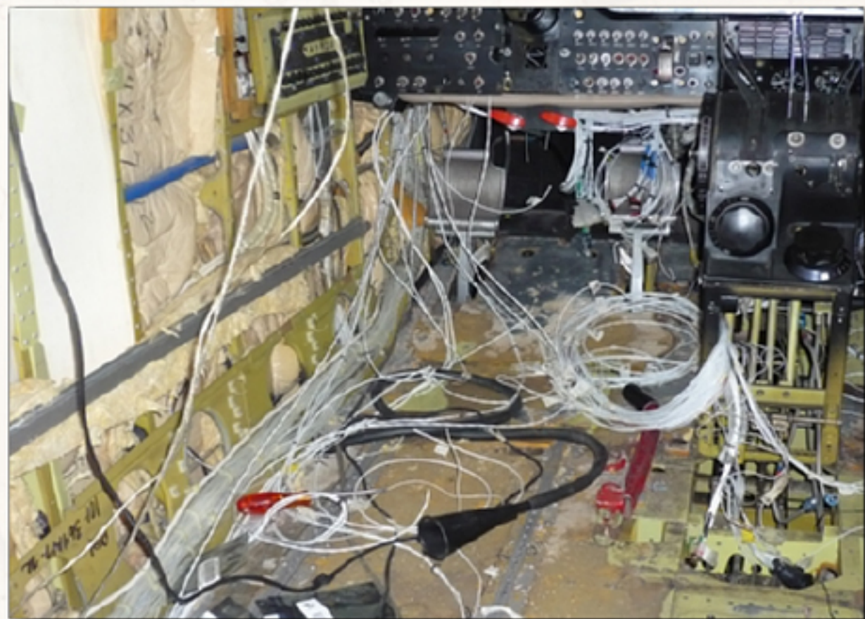
Removing old wiring
